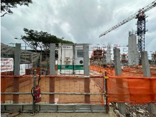
Picture 2: Battery Energy Storage System deployed at sites to reduce diesel consumption
